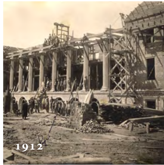
1912 - BATH WING UNDER CONSTRUCTION
