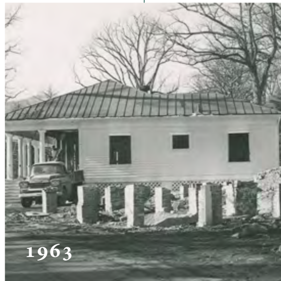
1963 – RENOVATIONS OF SOUTH CAROLINA F COTTAGE.
