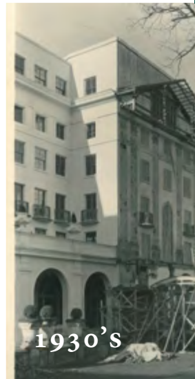
1930's - REPAIRS AND CONSTRUCTION OF THE HOTEL.
