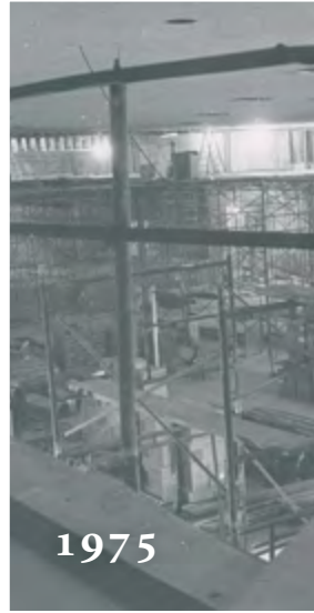
1975 – CONSTRUCTION OF COLONIAL HALL.
